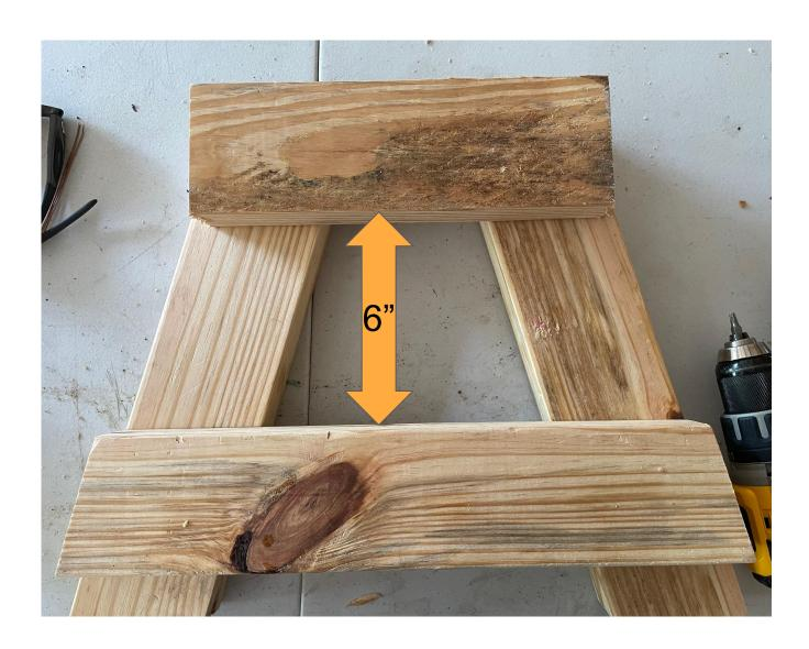
When attaching the bottom leg brace set it 6" from the bottom of the Top leg brace. Use 4 screws in each leg to attach the brace.
