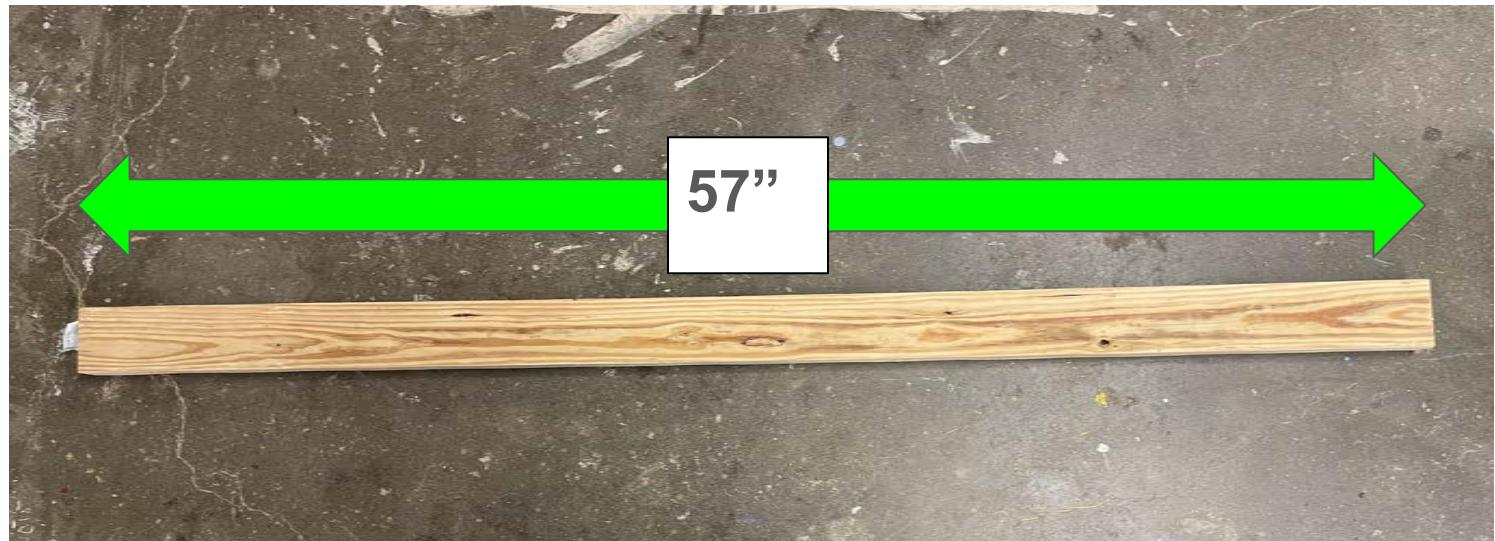
Cut three 57" long cross braces out of the treated 2x4s.
