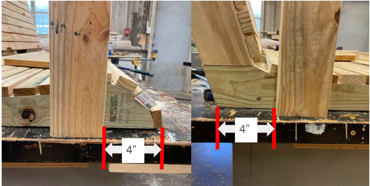
Cut from the 2x4 four 11" pieces for the arm rest supports. Position the front support 4" from the front of the seat. Then position the back support 4 inches from the bottom angle of the back of the seat brace. Secure with 2  $\frac{1}{2}$ " screws
