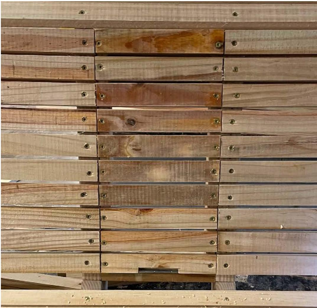
Install the slats on the front of the console gapping them a  $\frac{1}{4}$ ". Secure using 1  $\frac{1}{2}$ " screws. Recommend pre drilling holes for screws.
