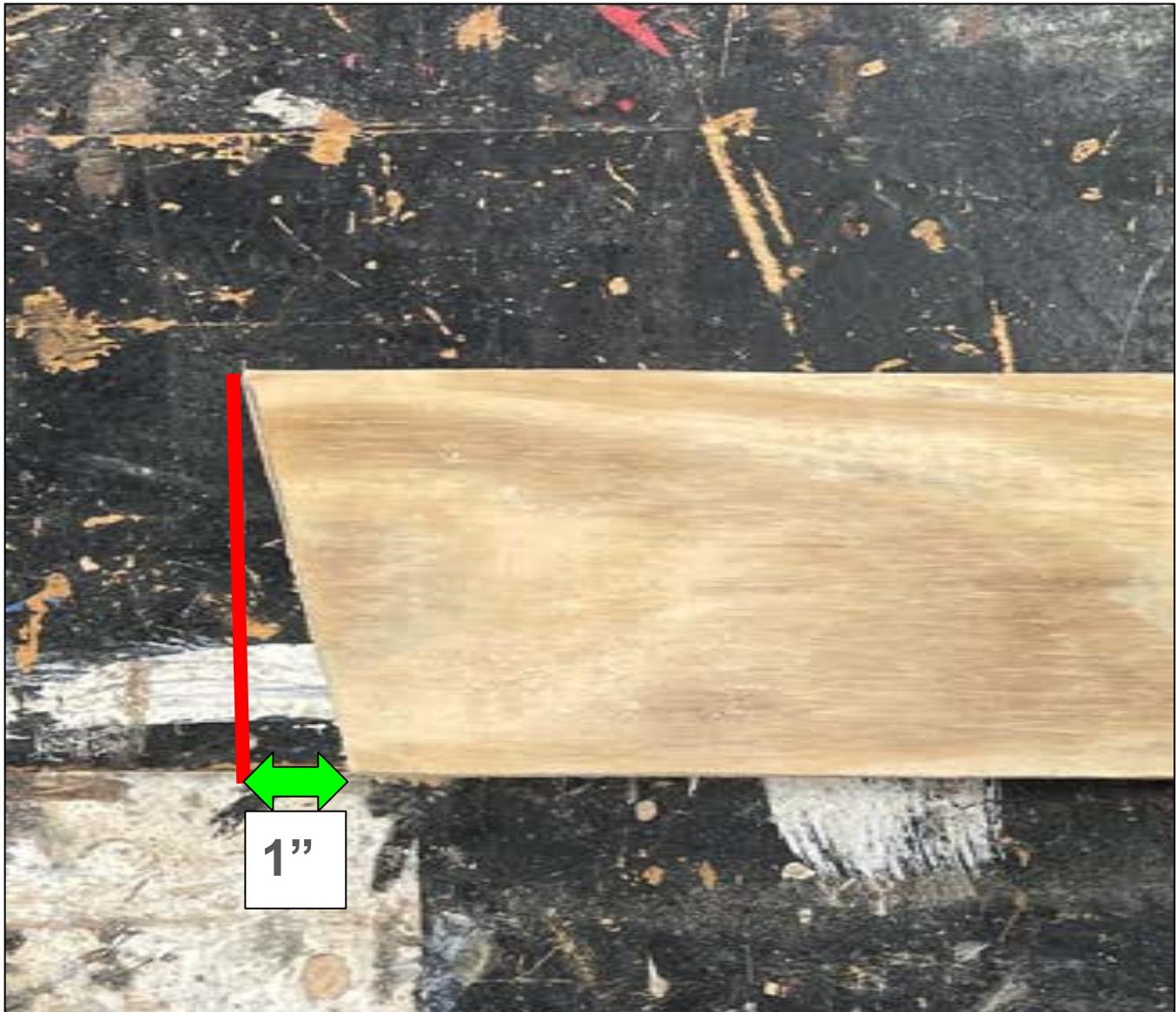
Next measure out 1" from the end of each 21" and 24" supports and then using a square draw a line to the adjacent corner then using a saw cut this angle on the end of each support.
