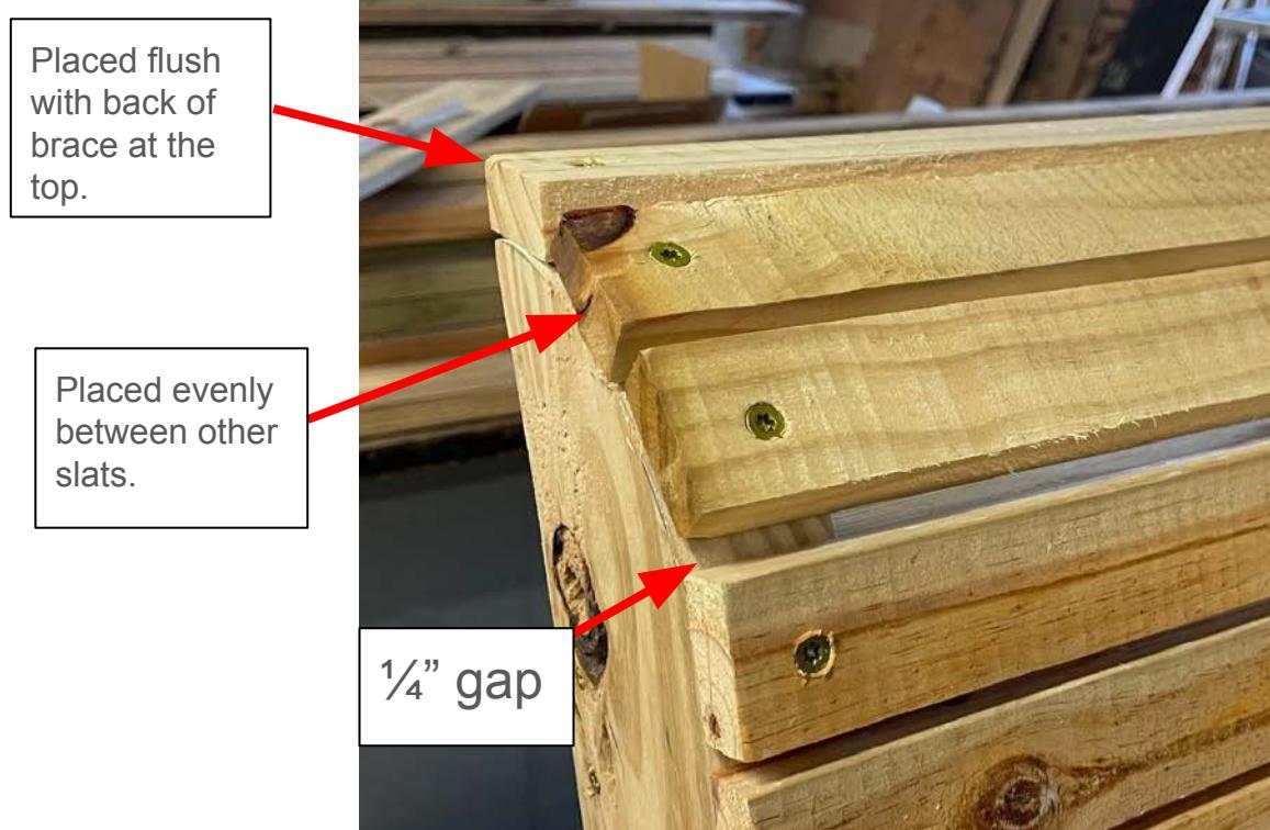
Cut the final 3 slats from the pre-ripped 1x2s 60" long for the top curve of the back brace. Install the first 60" right above the 25  $\frac{3}{4}$ " slats. Gap it  $\frac{1}{4}$ " from the 25  $\frac{3}{4}$ " slats. Secure with 1  $\frac{1}{2}$ " screws
