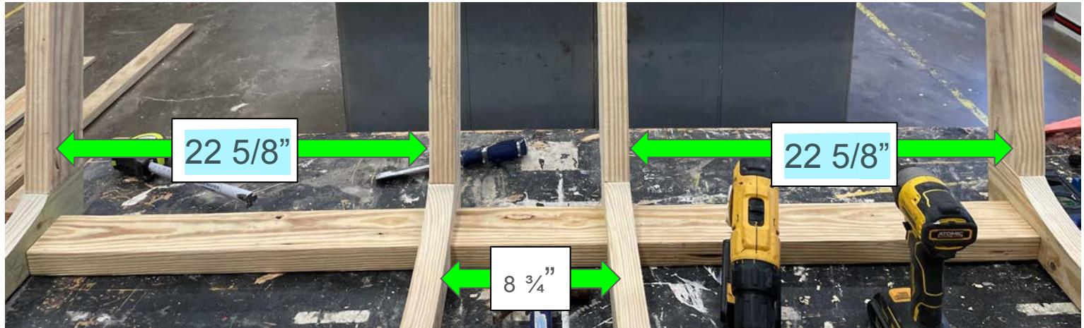
Take the middle braces with the cross brace slots and position them on the bottom cross braces and space according to the picture.
