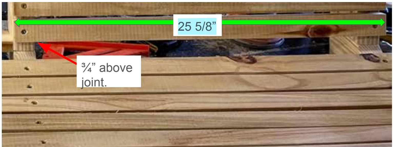
From the 1x2 ripped slats cut twenty 25 5/8" pieces. Place the first slat from the bottom above the 3/4" marks you made on the back braces and attach using 1 1/2" screws. Repeat this on the other side of the swing as well.
