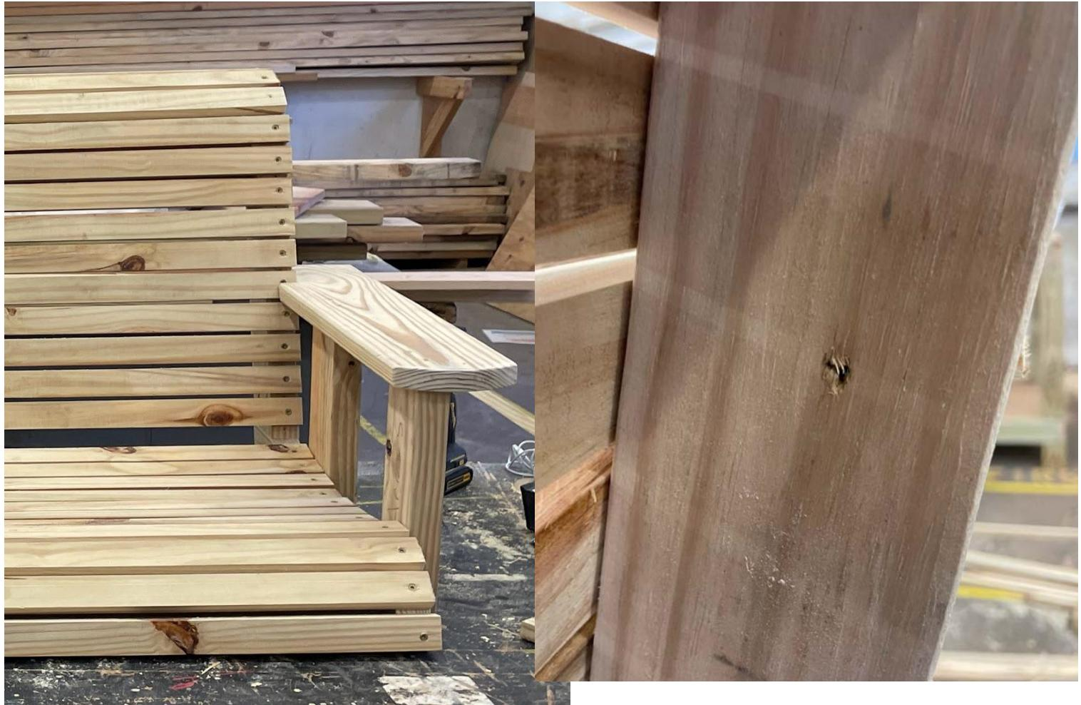
Install the arm using 2 ½" screws. Use two screws from top to attach the arm to the arm supports. Attach the notched end of the board with one 2 ½" screw from the inside of the end brace. Round the edges of the curved end of the arm rest.
