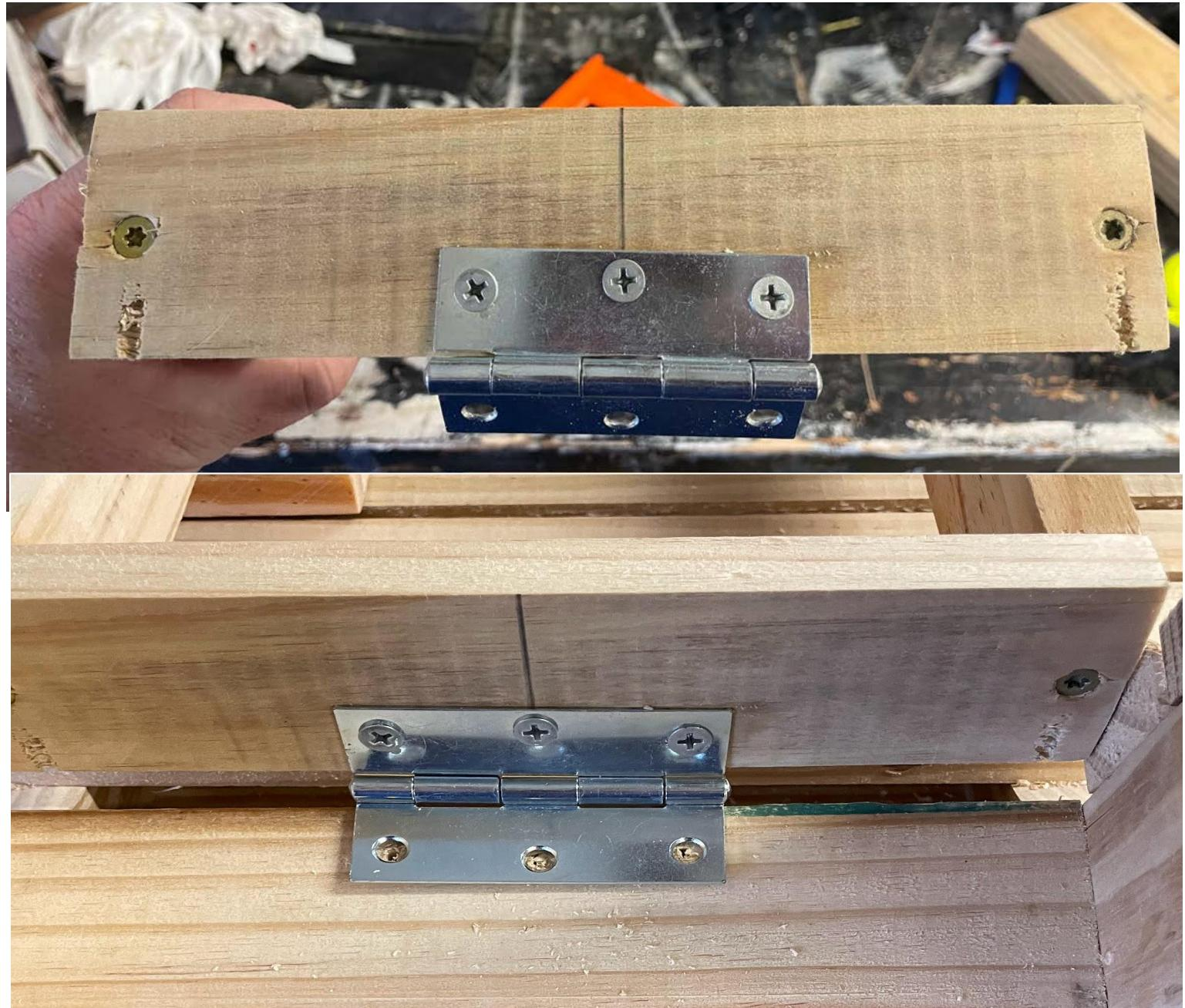
Take your 3" hinge and attach it in the middle of one of the 8  $\frac{3}{4}$ " sides of the frame. Then attach the other side of the hinge to the 1x4 console support.
