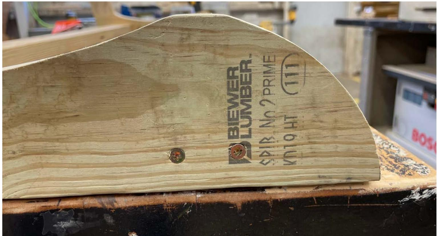
Attach from the outside of the brace using two 2 ½" screws on each side.
