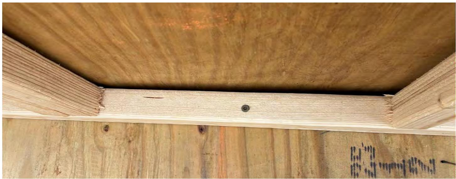
Line up the soleplate of the front wall assembly on the floor assembly and secure the soleplate to the floor using at least 5-3" screws evenly spaced.
