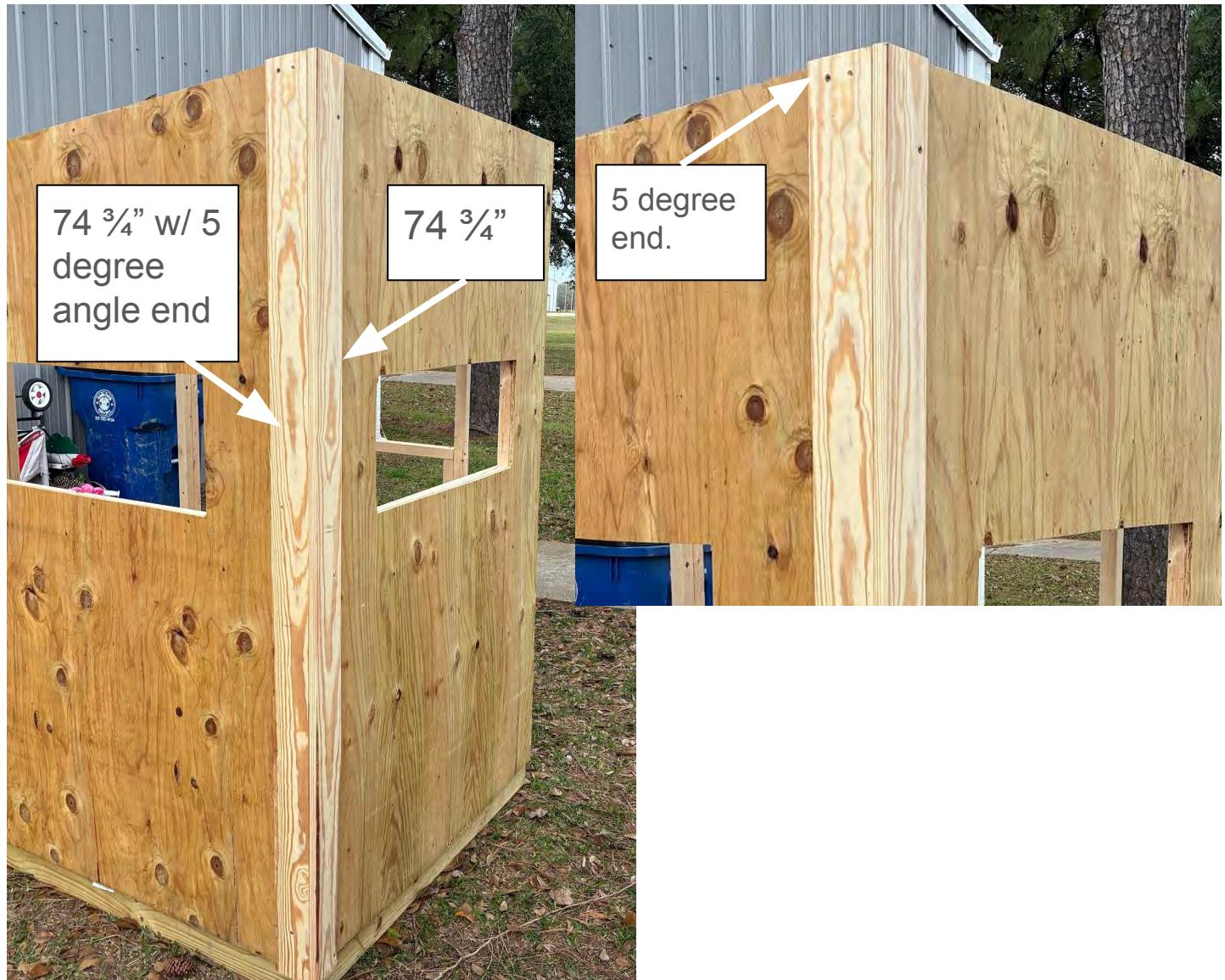
Cut 1-  $74 \frac{3}{4}$ " piece from your treated 1x4s that has a square cut on both ends.
