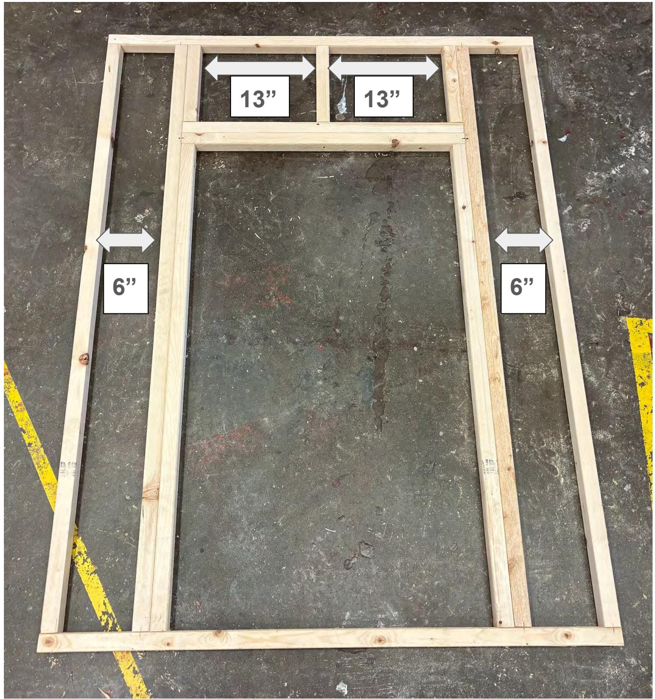
Layout boards according to these gaps and attach boards together using 3" and 2" screws. The 5 degree angled side of the precut 48" top plate should be faced up when installed.
