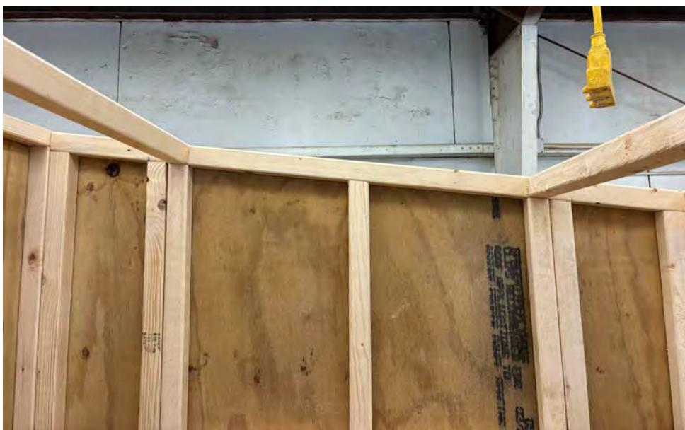
Cut 2-45" roof braces from your 2x2s and attach them using 3" screws above the first and third crippler studs as shown in the diagram.
