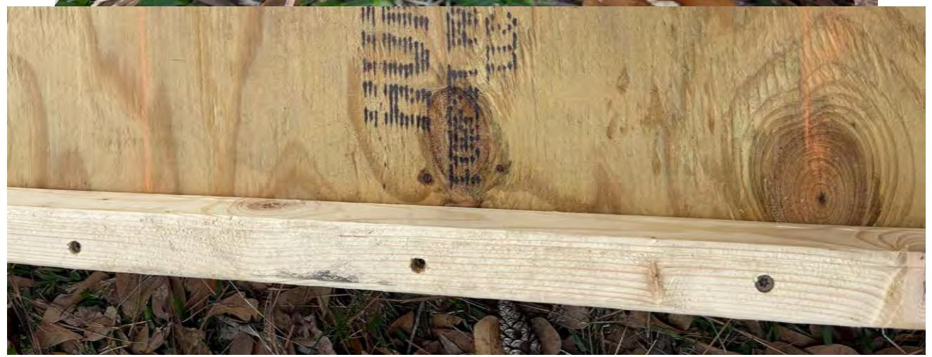
First Take the back wall assembly and line it up with the edge of the floor assembly. Attach the back wall assembly to the floor assembly using no less than 5-3" screws spaced out evenly.
