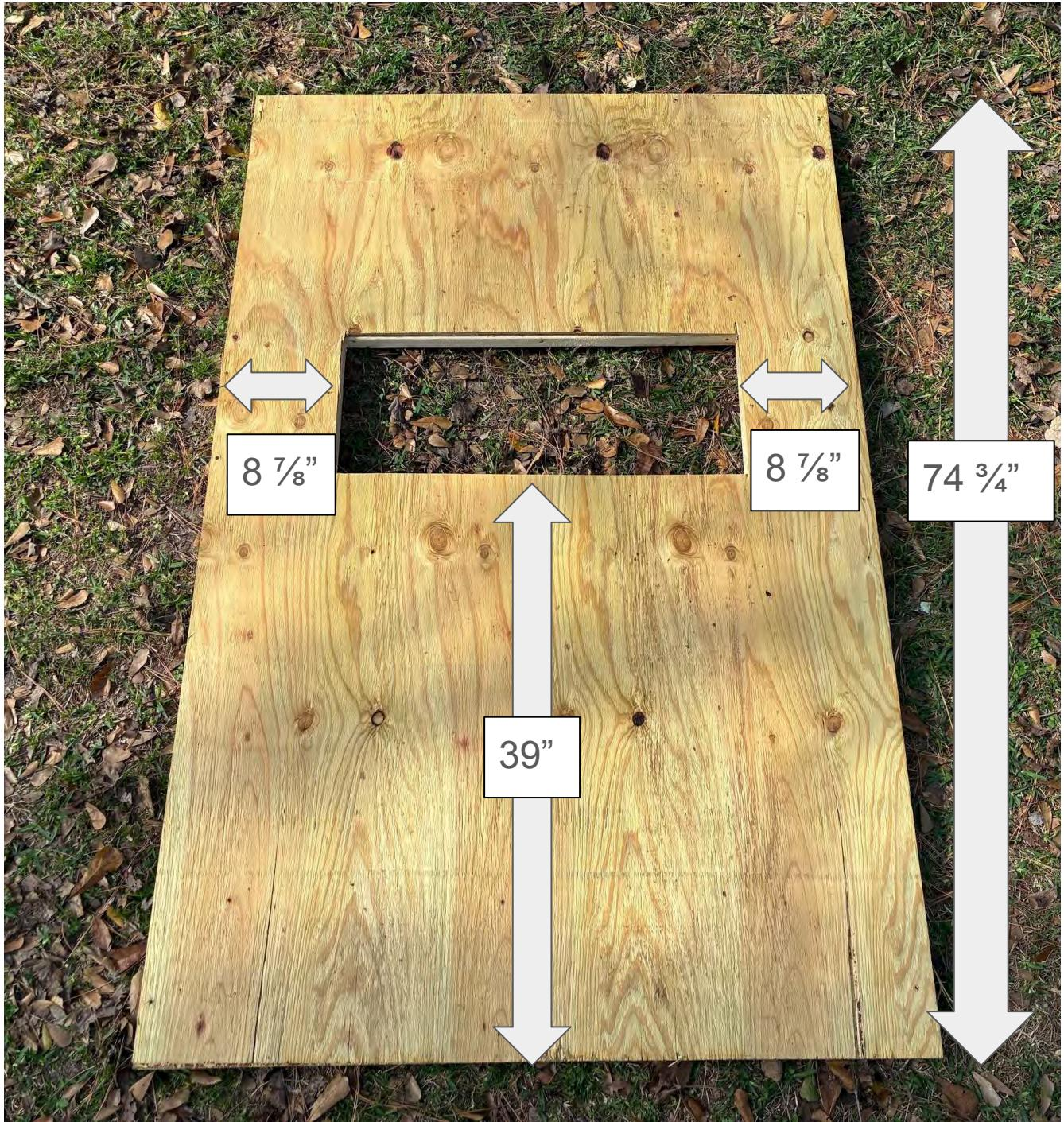
Take one sheet of your  $\frac{3}{8}''$  Treated plywood and cut the sheet according to the above specifications for the front wall assembly.
