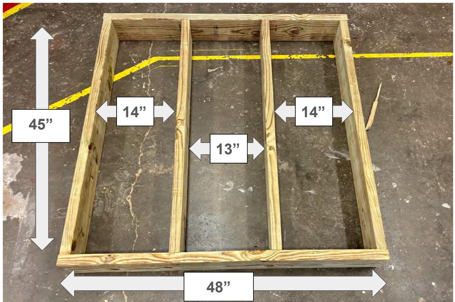
Layout your floor assembly according to the diagram and attach together with 3" screws.
