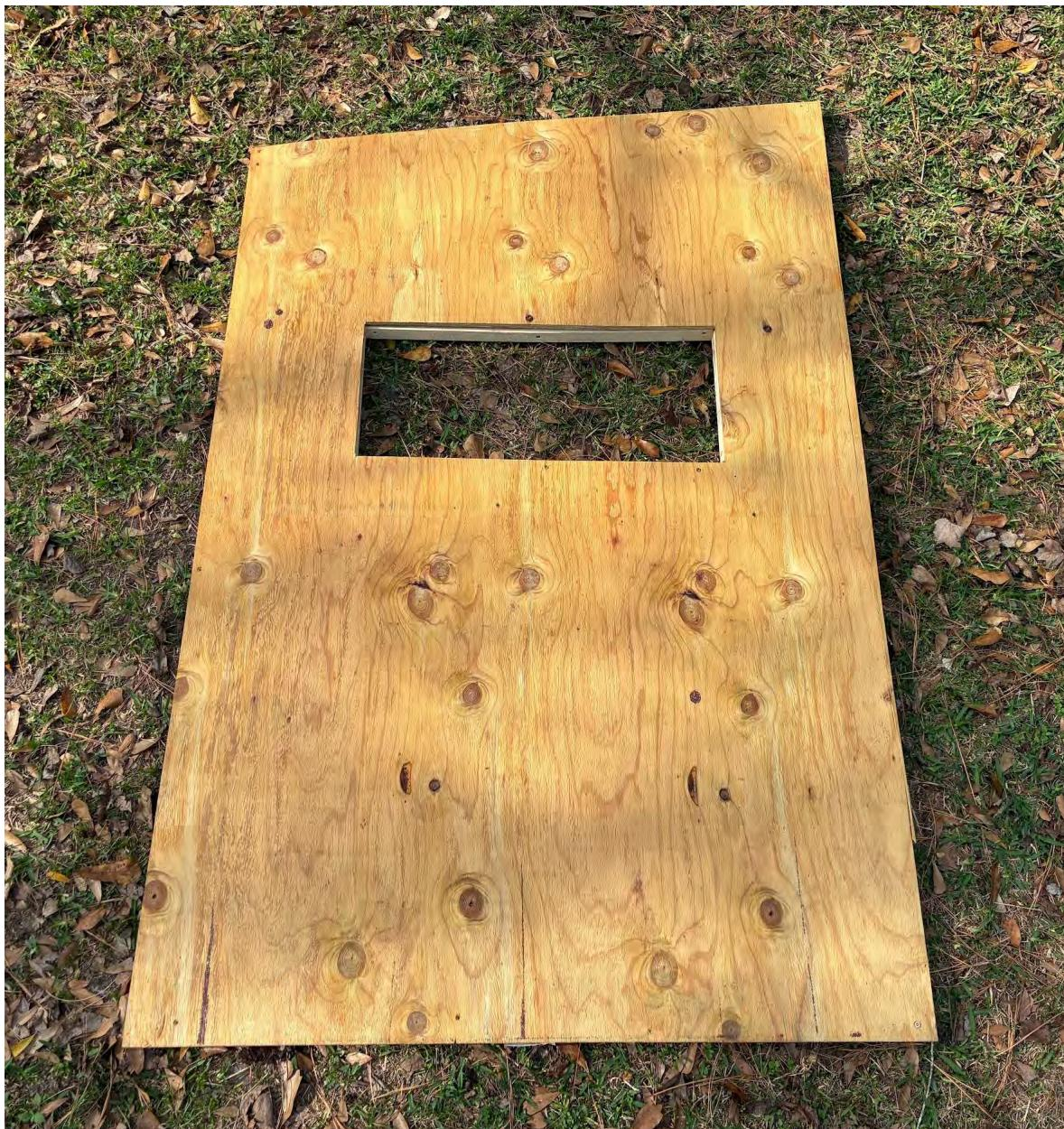
Align the sheathing for the right wall assembly by lining up window with the window frame and with the top plate. Attach sheathing using 2" screws.
