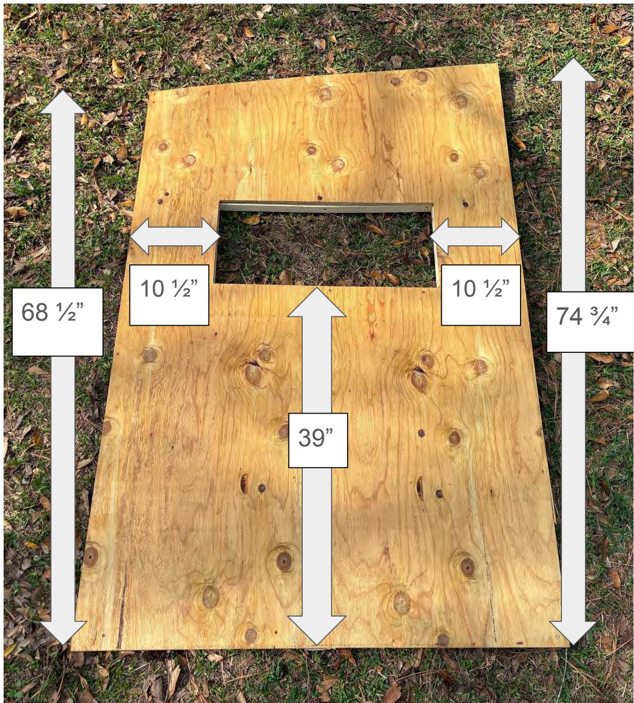
Take the other sheet of your  $\frac{3}{8}''$  Treated plywood and cut the sheet according to the above specifications for the right side wall assembly.
