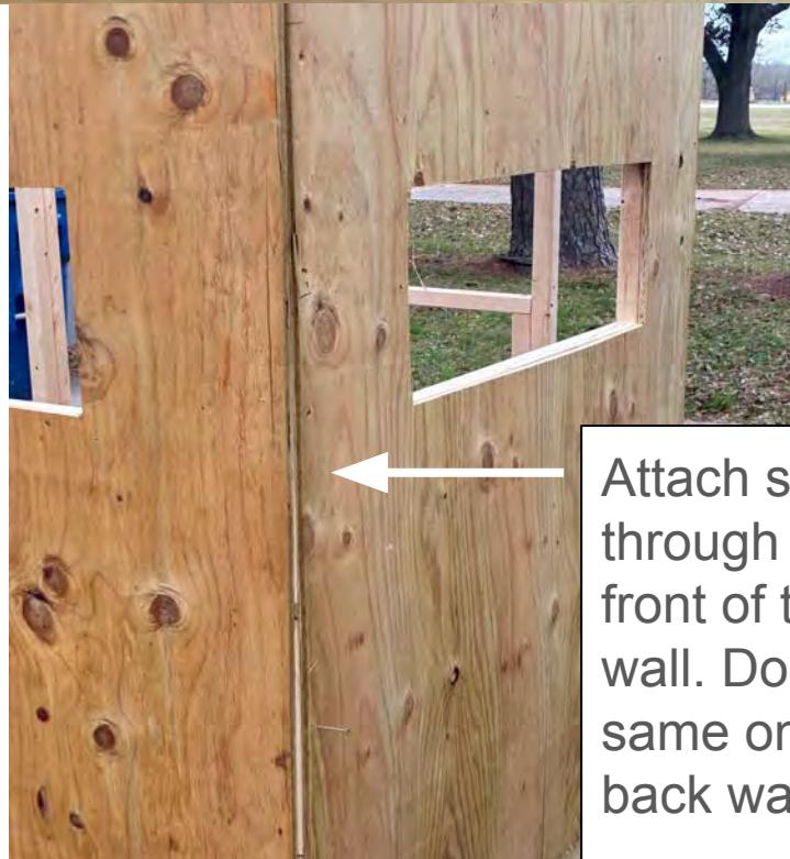
Attach wall to the floor assembly using no less than 5-3" screws spaced evenly. Attach the corner of the side wall to the back wall and front wall by using no less than 5-2 1/2" screws driven from the front a back wall side spaced evenly.
