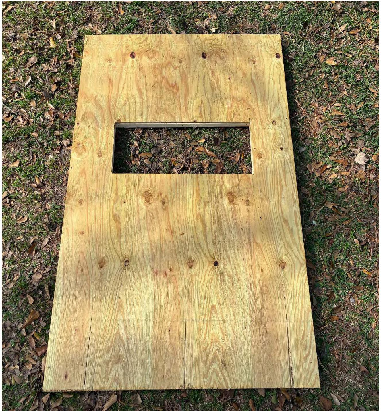
Lay Sheathing for the front wall assembly on top on top of the assembly and line up the top corners and sides. Install on the wall assembly using 2" screws.
