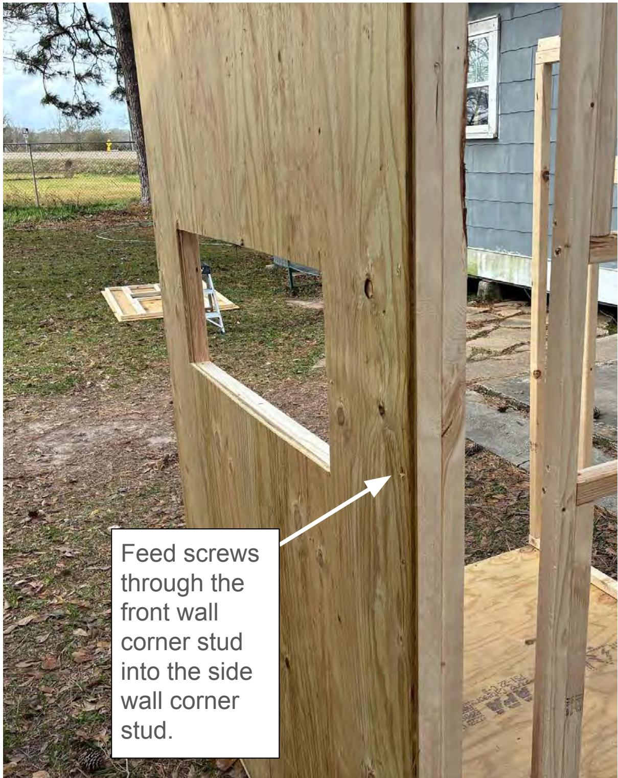
Using at least 5-3" screws attach the corners of the front and side wall assemblies from the outside of the plywood. Space screws evenly.
