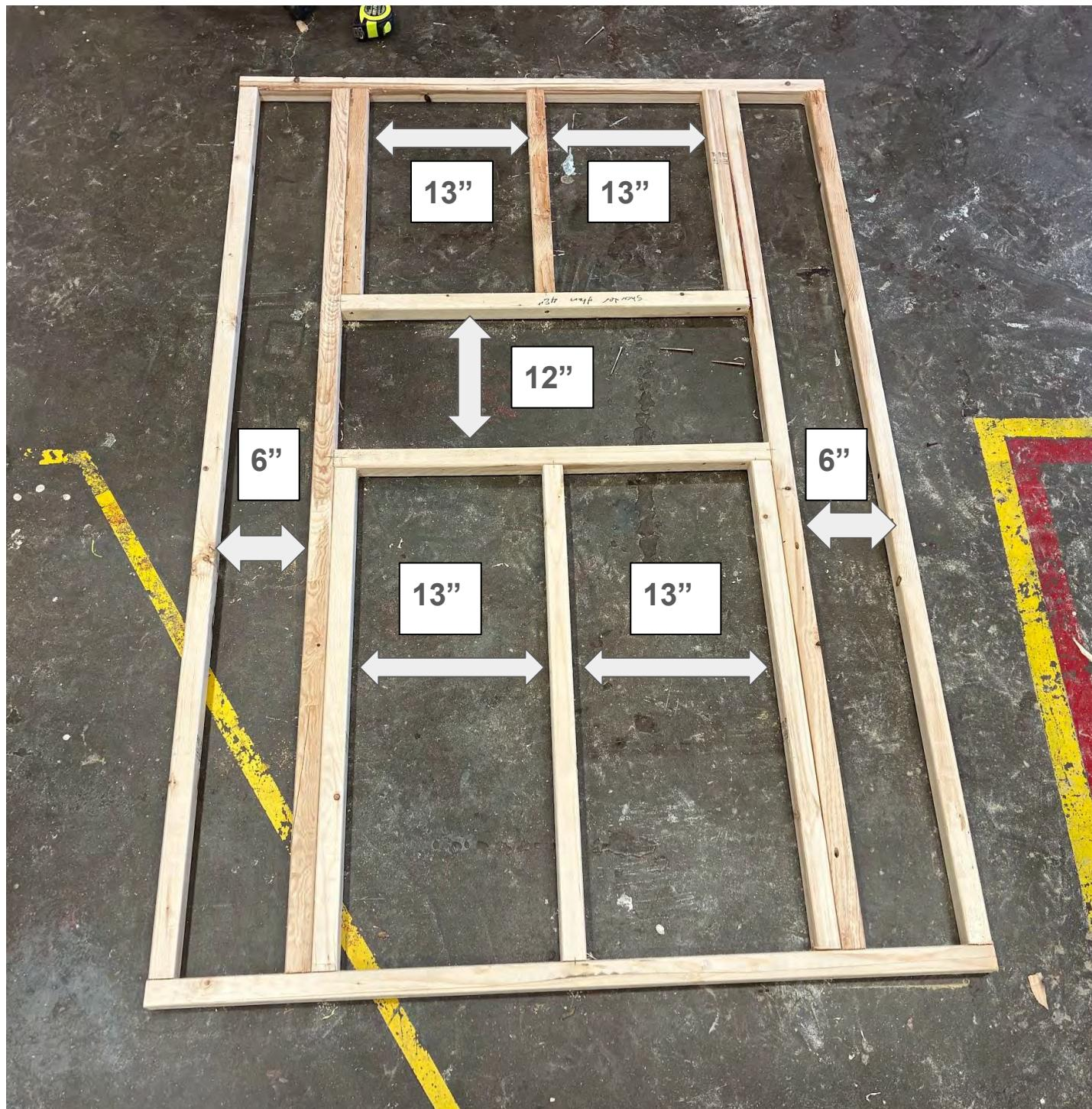
Layout boards according to these gaps and attach boards together using 3" and 2" screws. The 5 degree angled side of the precut 48" top plate should be faced up when installed.
