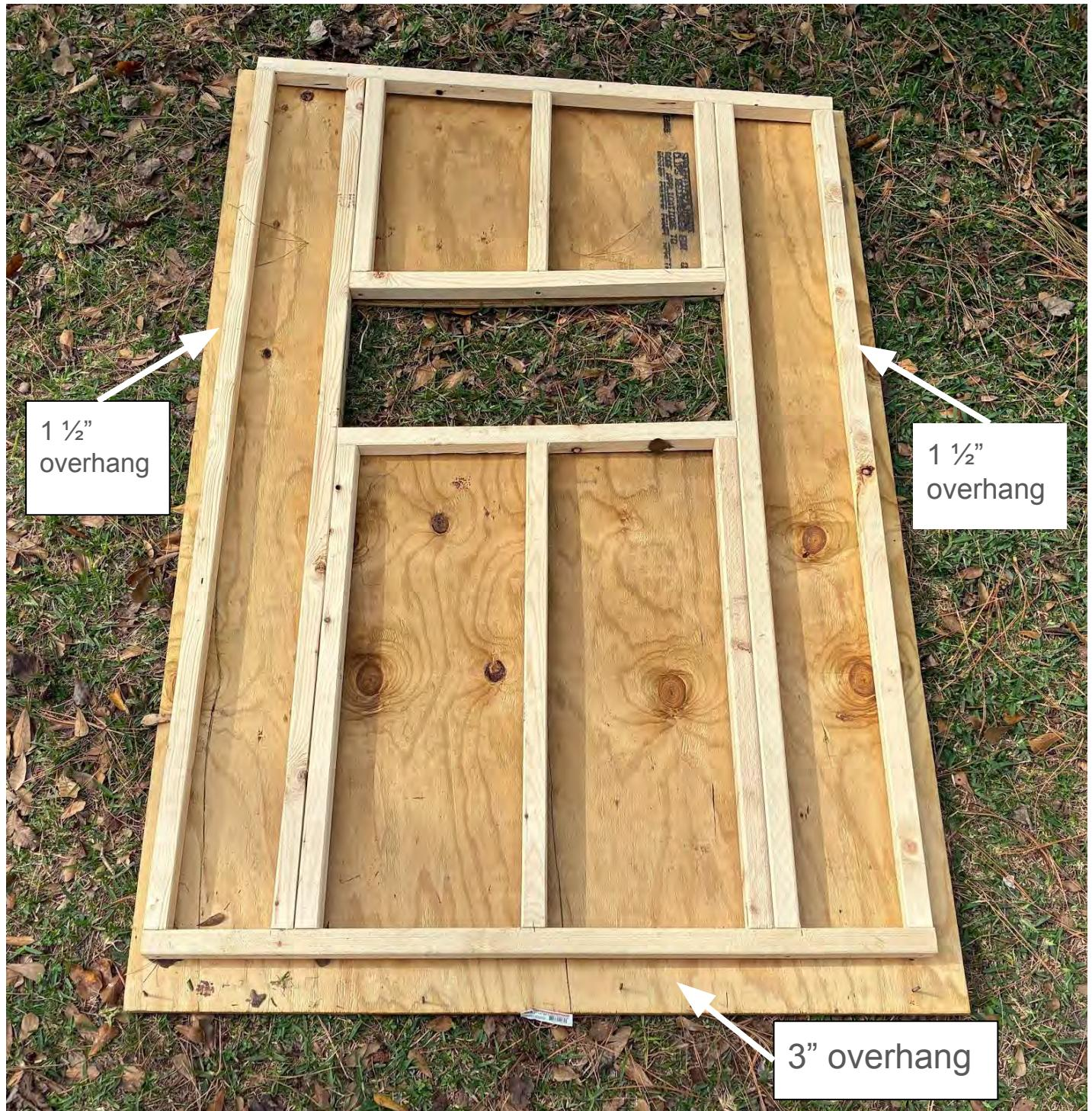
You should have a 3" overhang on the bottom of the wall assembly and a 1 1/2" overhang on each side of the assembly.
