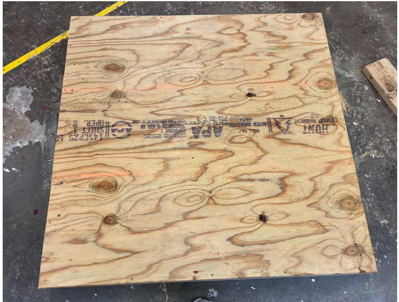
Take your cut out Subfloor and attach it to the floor assembly using the 2" screws.
