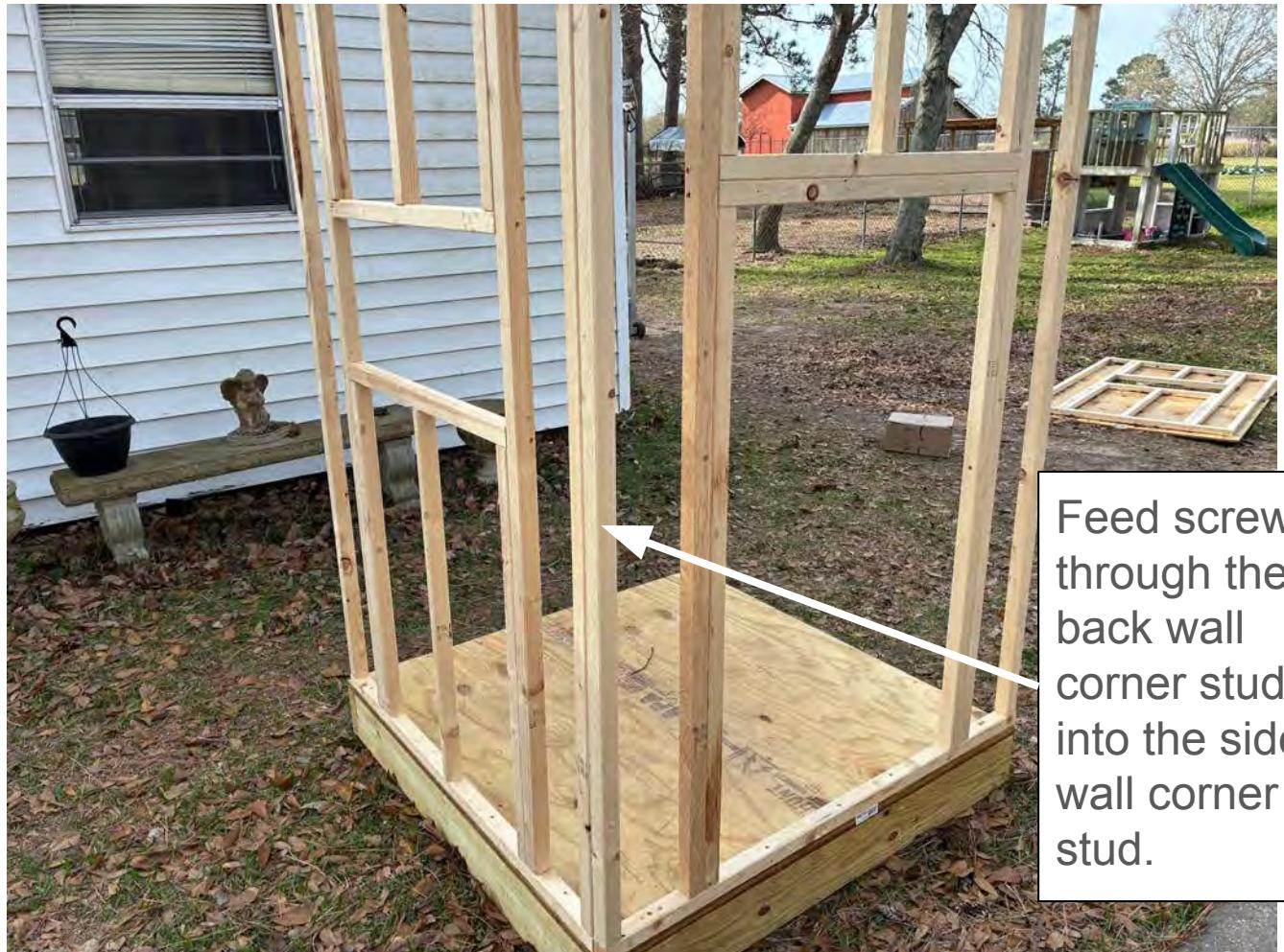
Feed screws through the back wall corner stud into the side wall corner stud.
