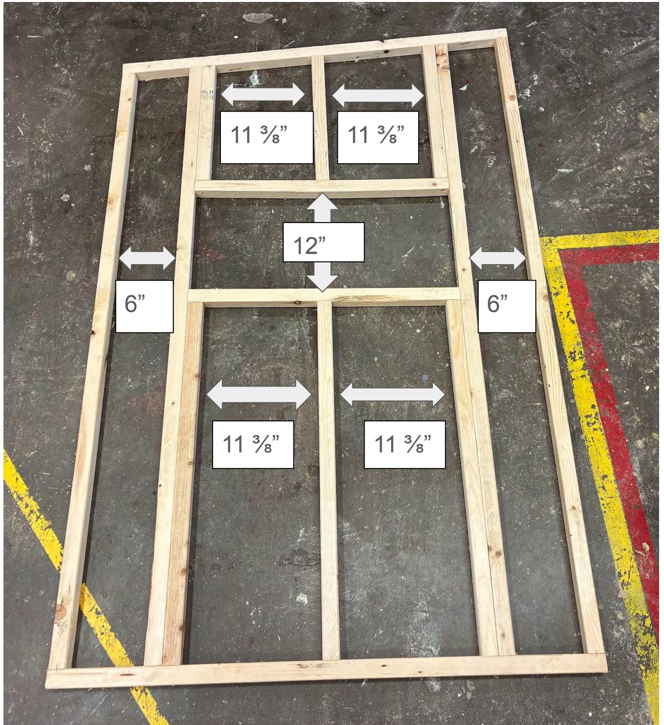
Layout boards according to these gaps and attach boards together using 3" and 2" screws. The 5 degree angled side of the precut 48" top plate should be faced up when installed. Follow the same pattern for both side walls
