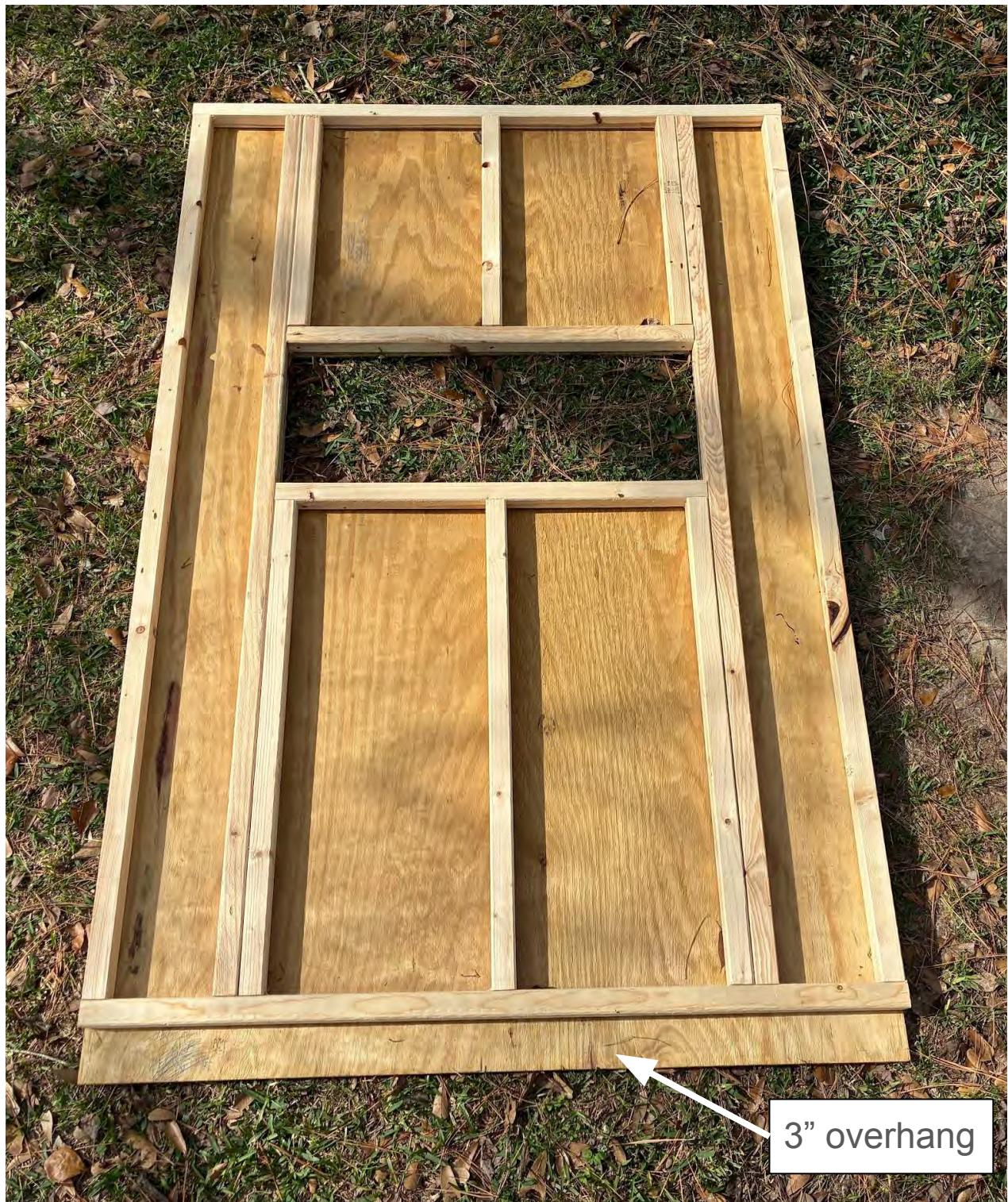
You should have a 3" overhang on the bottom of the wall assembly.
